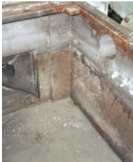
Corrosion in the resevoir
